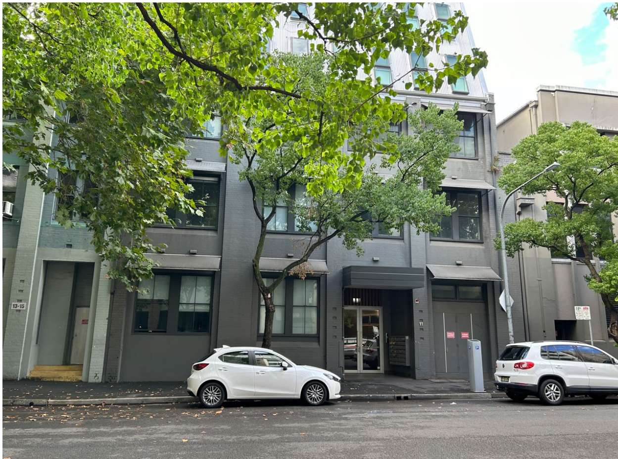
Neighbouring residential flat building (11 Smail Street, Ultimo)
